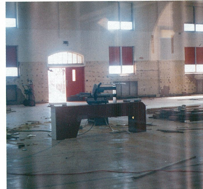
Construction gets underway in the old gym.
